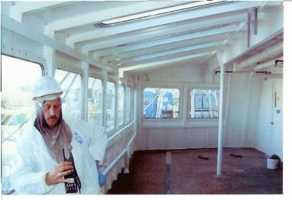
A West Coast Insulation coatings professional checks coatings thickness. With two passes totaling 40 mils (DFT), Mascoat Delta dB provided enough acoustic insulation to ensure hovercraft passengers and crew would not be forced to wear earplugs while underway.
